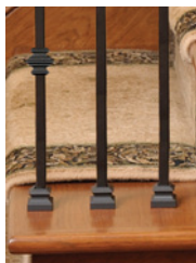
Open Tread Bottom Connection
